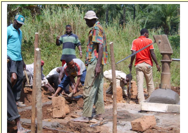
Repairs to an existing well
