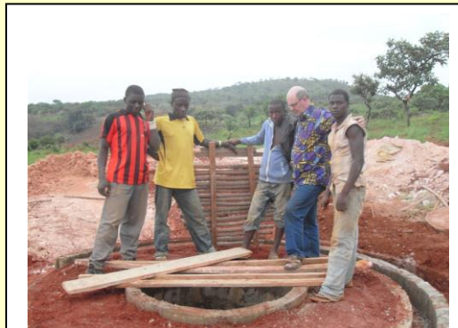
A new well under Construction
