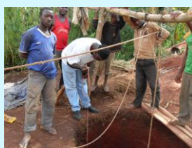
Measuring the depth of a new well.....
