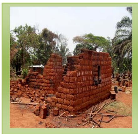
A home destroyed in Bambalang
