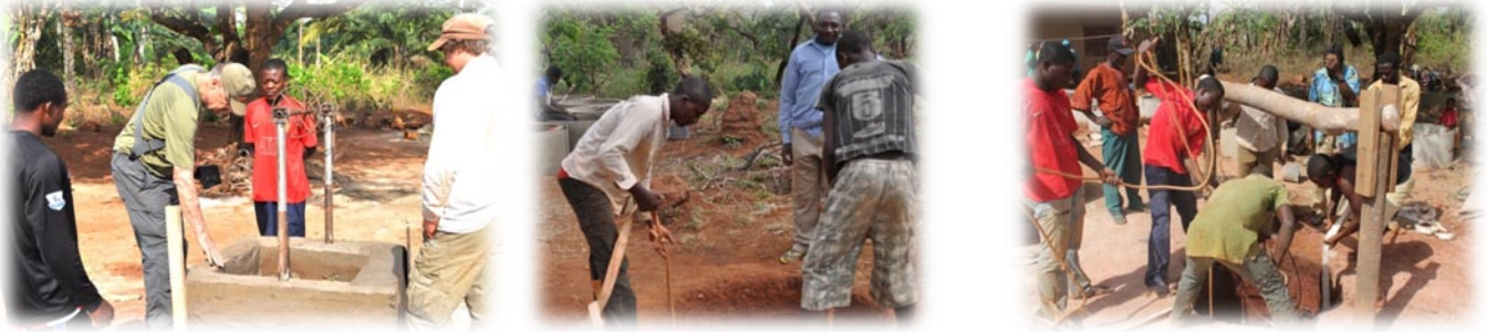
The Type B Well at Ngwalla under construction. This well is more than 22metres deep. All dug by hand.
