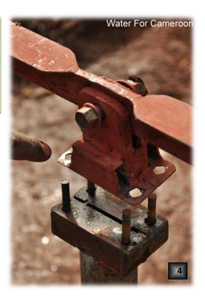
Photo No. 4 The pump handle is fixed to the pump stand. We do have a pump stand and handle made from wood that will be trialed at a later stage.
