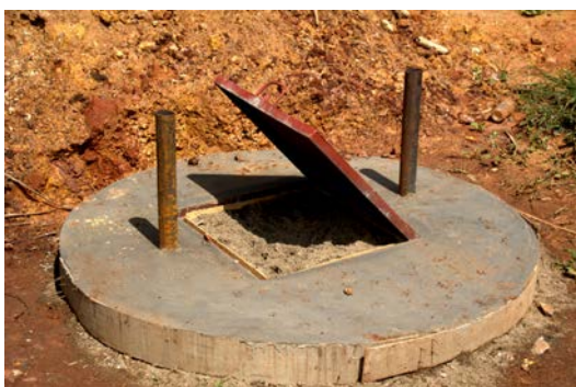
The Lid for the Well is prepared
