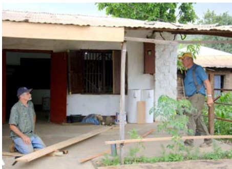
Don & Jerry work on repairs at The Water Shop
