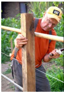
Jerry works on the fence at The Ndop Water Shop
