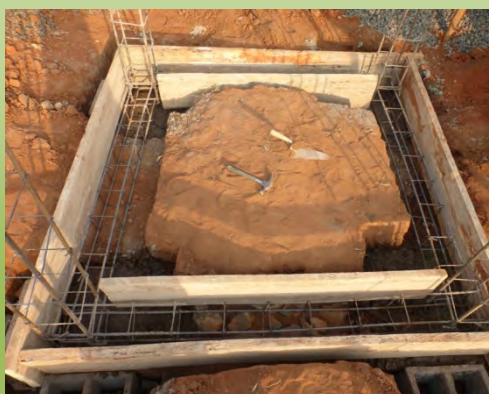
Water tower foundations are prepared for Concrete to be poured.
