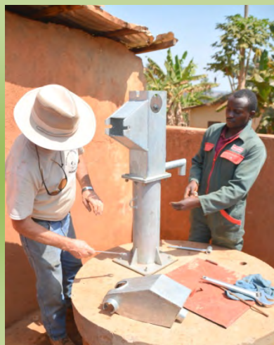
Don Williams and Ambe work on fitting an Afridev pump to an existing Well in a primary school in Bambalang in December 2015.
