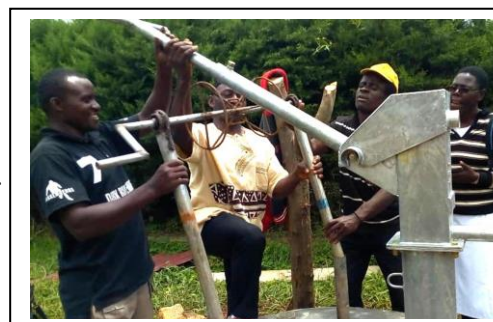
Futura Well at Bamenda
