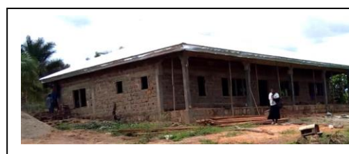
The new clinic under construction
